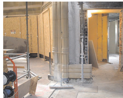
Cast concrete stones in Suzzallo Reading Room. Photo by Paula Walker.
