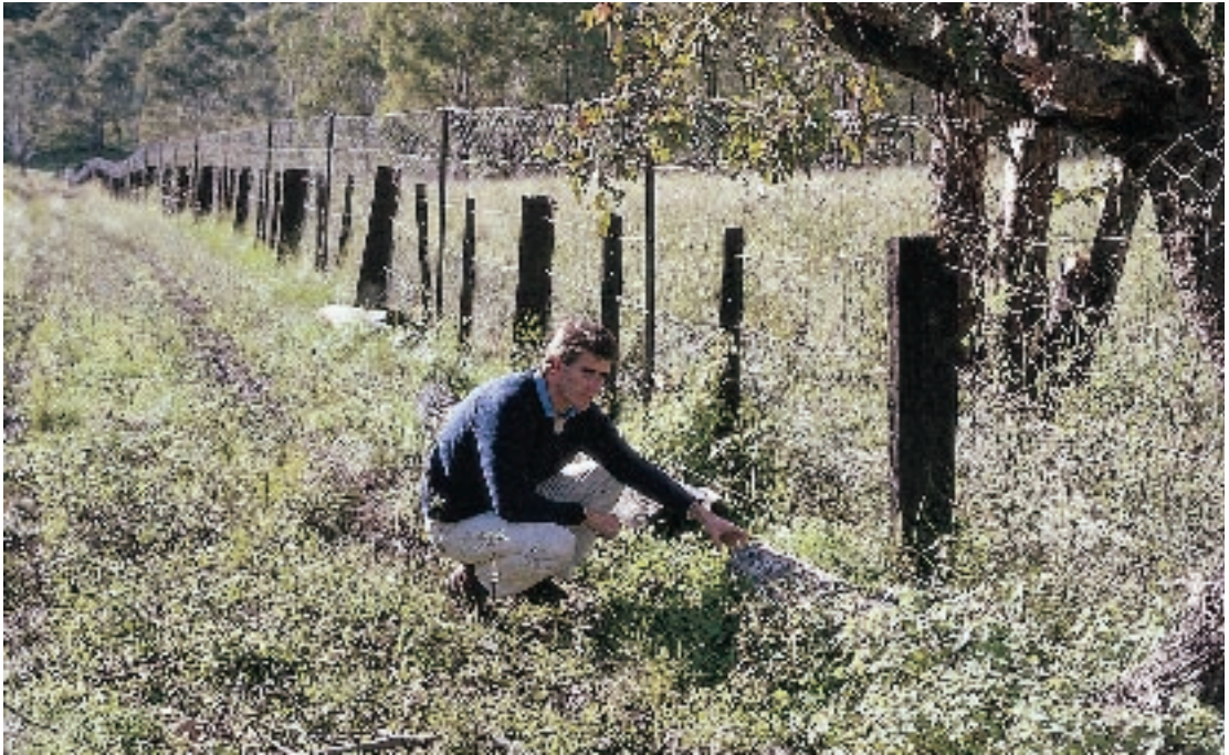
Figure 12: A wire-netting wild dog-proof fence in north-eastern New South Wales. The fence has a single electrified outrigger wire and logs placed at the bottom to prevent damage by macropods (Source: P. Fleming).
